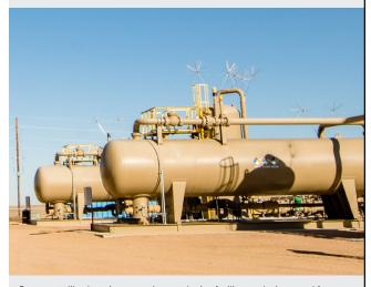
Separators, like these in a natural gas gathering facility, can be inspected for gas leaks and checked for efficient operation.
